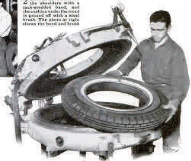
4 NEW RUBBER BONDED ON BY VULCANIZING As the final process, the new tread is vulcanized to the body in a steam-jacketed curing mold. The new rubber fills the spaces between the cords and forms a perfect bond. The tire is now ready for use.
